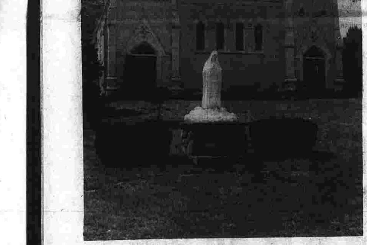
St. James Church, 38 years apart. The steeple was toppled by the hurricane of Sept. 21, 1938, and the heavy bell crashed into the building below, causing heavy damage to the south end of the church. (Herald photo by Bucevicius)
